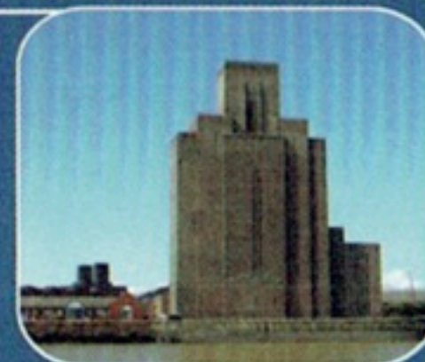
Queensway Tunnel Ventilation Station Built in the Art Deco style designed to pump fresh air to the roadway below.
