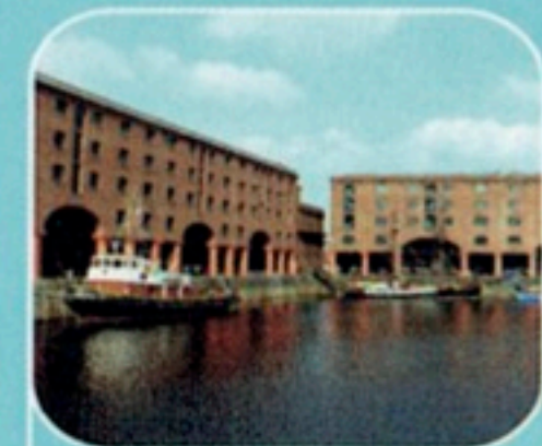
Royal Albert Dock Opened in 1846. The first structure in Britain to be built from cast iron, brick and stone.
