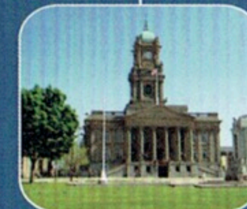
Birkenhead Town Hall Opened in 1887, it was built using local Sandstone from Storeton quarry and Scottish Granite.
